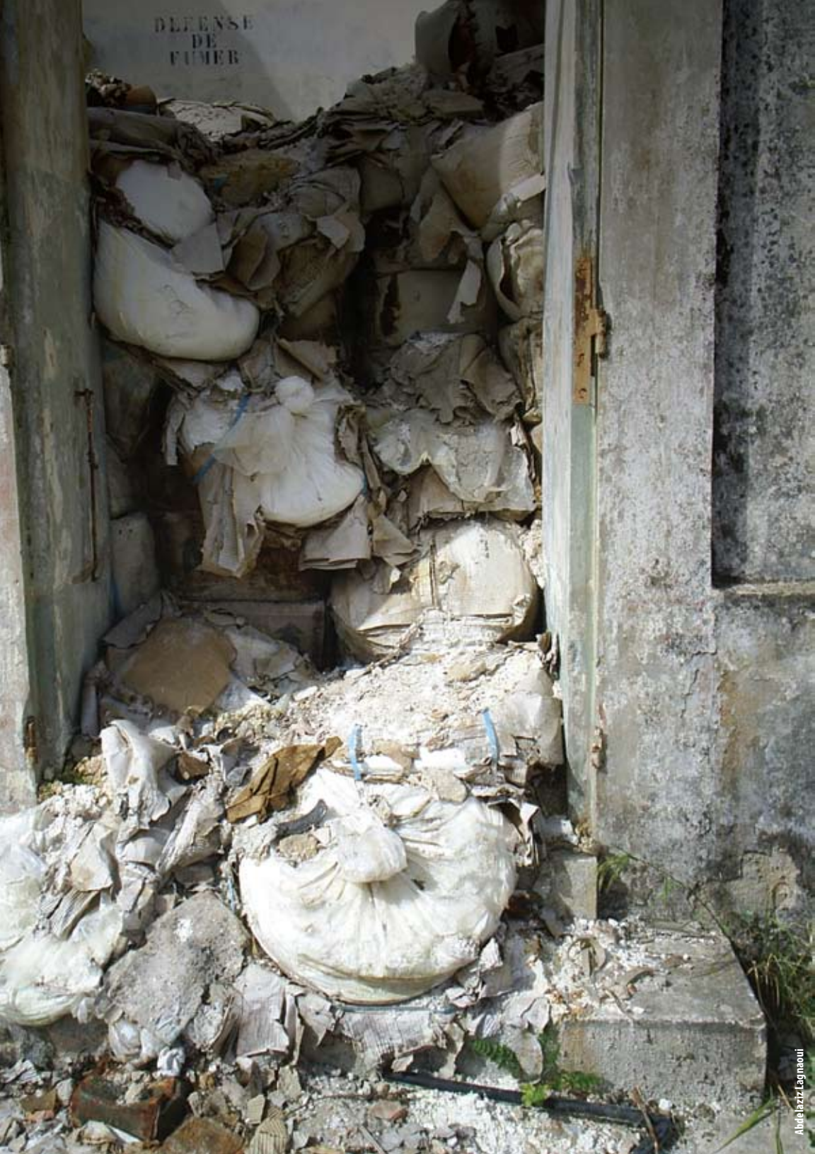
An old DDT storage facility in the Regional Hospital of Menzel Bourguiba, Tunisia.
